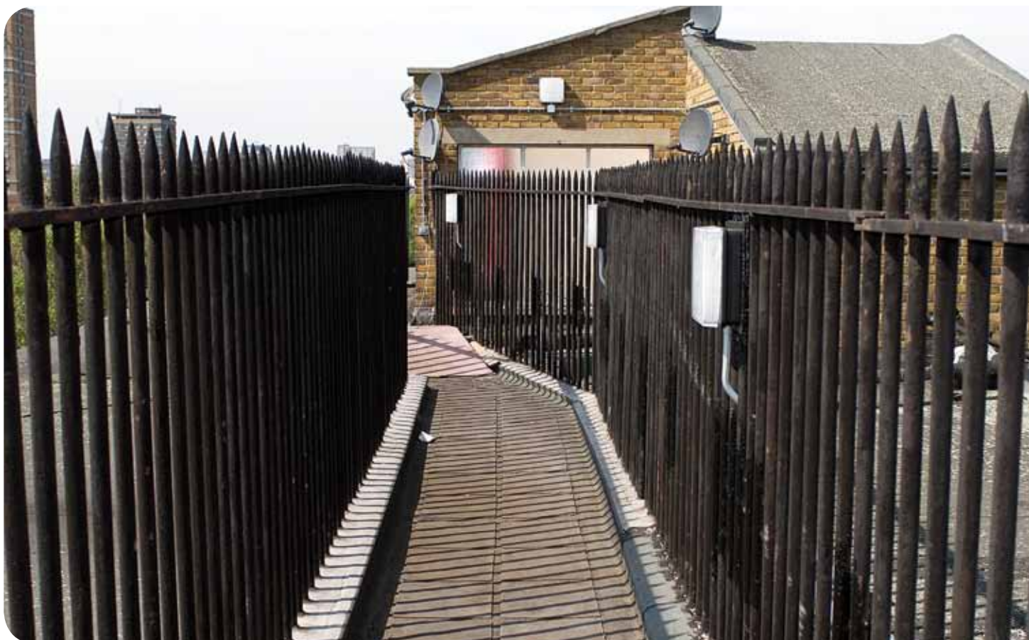
Figure 11 – Protection to an external stairway
