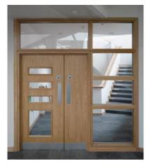
Fire doors are an essential part of a building's Passive Fire Protection, ensuring that the building is compartmentalised and helping to prevent the fire from spreading, allowing any occupants time to escape.
